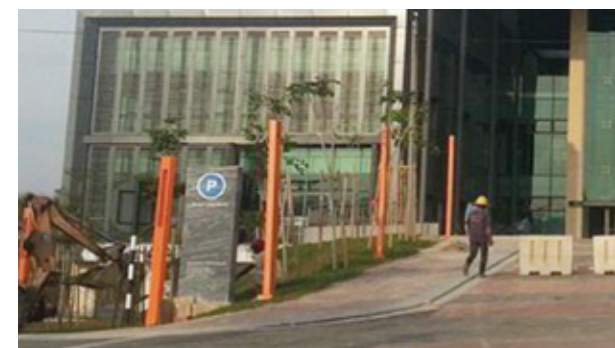
Blok Pentadbiran / Administration Block.
