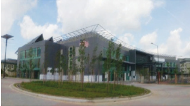
Blok Pentadbiran / Administration Block
